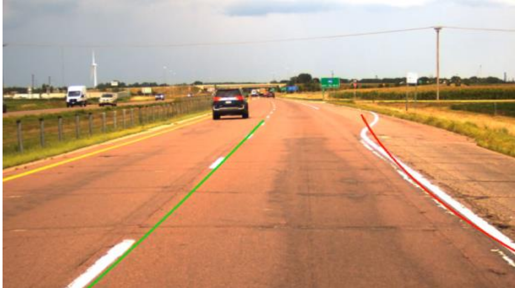
Figure 16 - Misdetection of Lane Due to Unstriped Diverge Area
