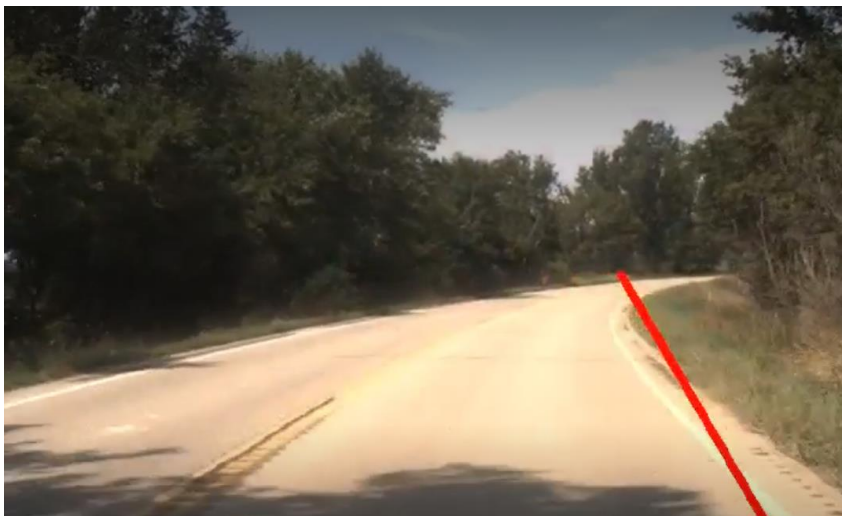
Figure 27 - Especially Sunny Area Makes Marking Indistinguishable
